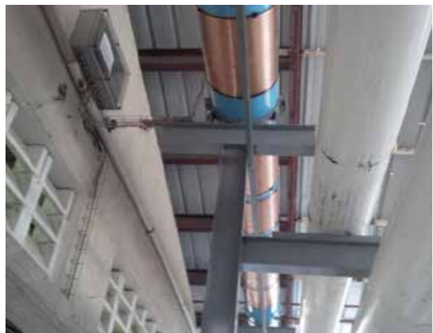
Vulcan S500 cable windings
